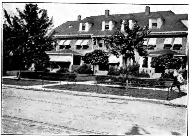
A SUCCESSFUL ATTEMPT AT MAKING A THREE-FAMILY HOUSE ATTRACTIVE Houses in Cleveland, Ohio.
